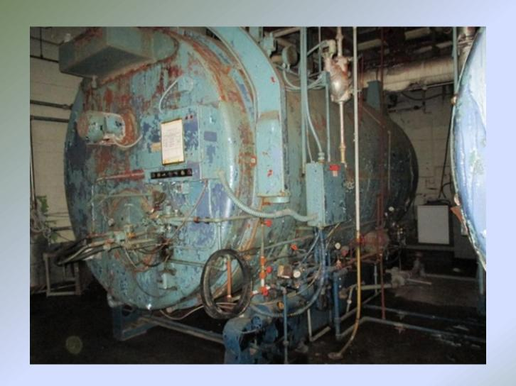
Cleaver Brooks 350 High Pressure Steam Boiler with Piping and Electrical Controls
