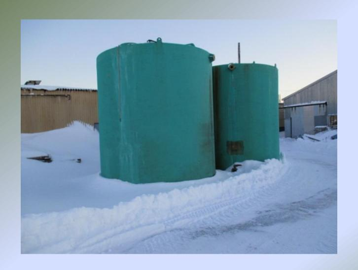
Fiberglass Tank 4 ft. x 8 ft. 44 in. High with Piping and Structure Support
