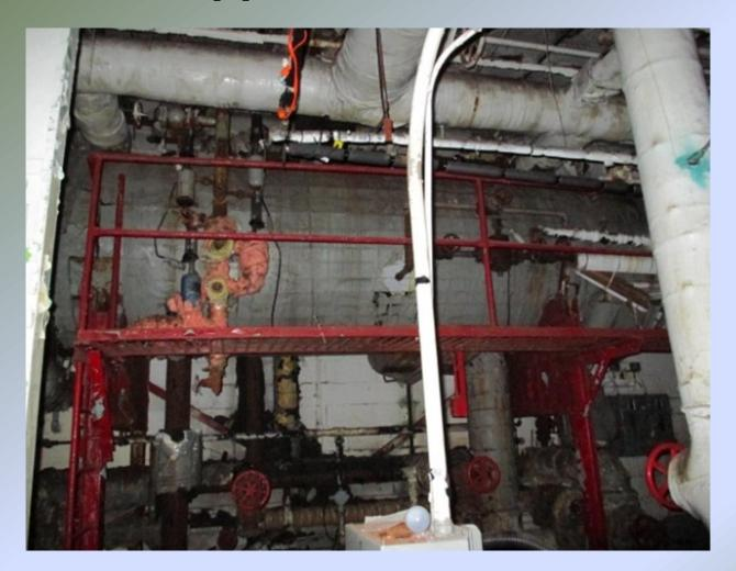
Ammonia Low Pressure Receiver 2 ½ ft. Diameter x 12 ft. Long with Piping and Valves
